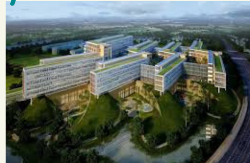
Shanghai Eastern Hepatobiliary Hospital
